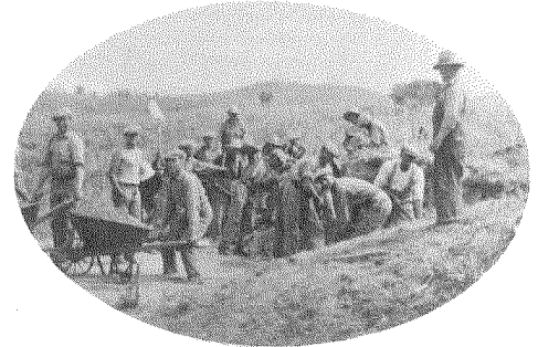
Digging a filling on a spur, Dundurn, Saskatchewan
