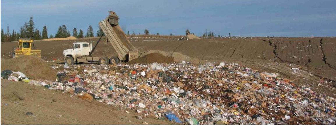
Figure 22: Compacted garbage is ready for a cover of soil. The dumped soil will be spread across the garbage to create a refuse cell. The soil-covered slope in the background is underlain by many refuse cells.
