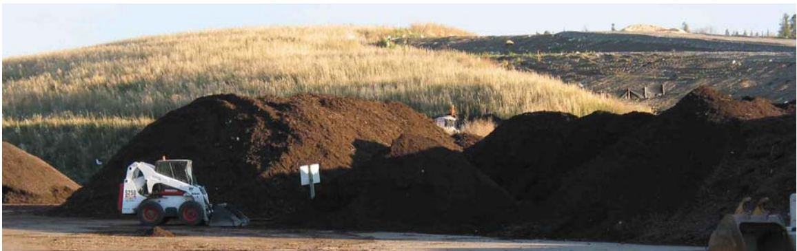
Figure 23: Composted greenwaste piles (brown, foreground) will be used as a soil amendment. After the landfill has been covered with soil (right, background) it is seeded with grass (left, background)
