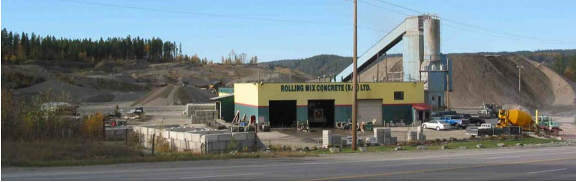
Figure 13. Concrete plant and sand-gravel quarry on Foothills Boulevard. Sand and gravel are quarried from the forested flat-topped bench (an ancient river plain) in the background.
