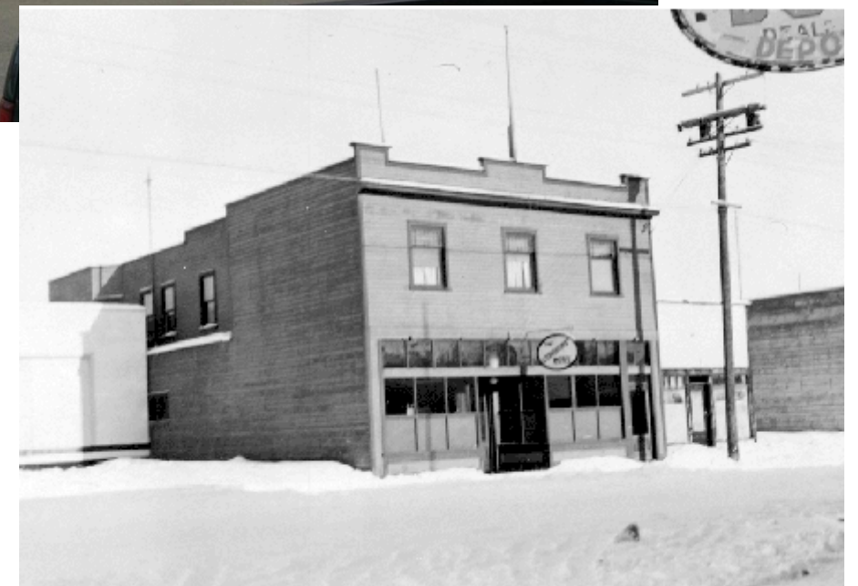
Figure 14: The Croft Hotel (formerly the Corning - see inset), is recognized by many Prince Georgians as an important historic place. It represents a significant part of the city's twentieth century development.
